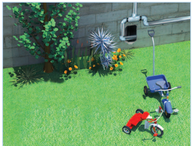
Openings are entrances for pests.
